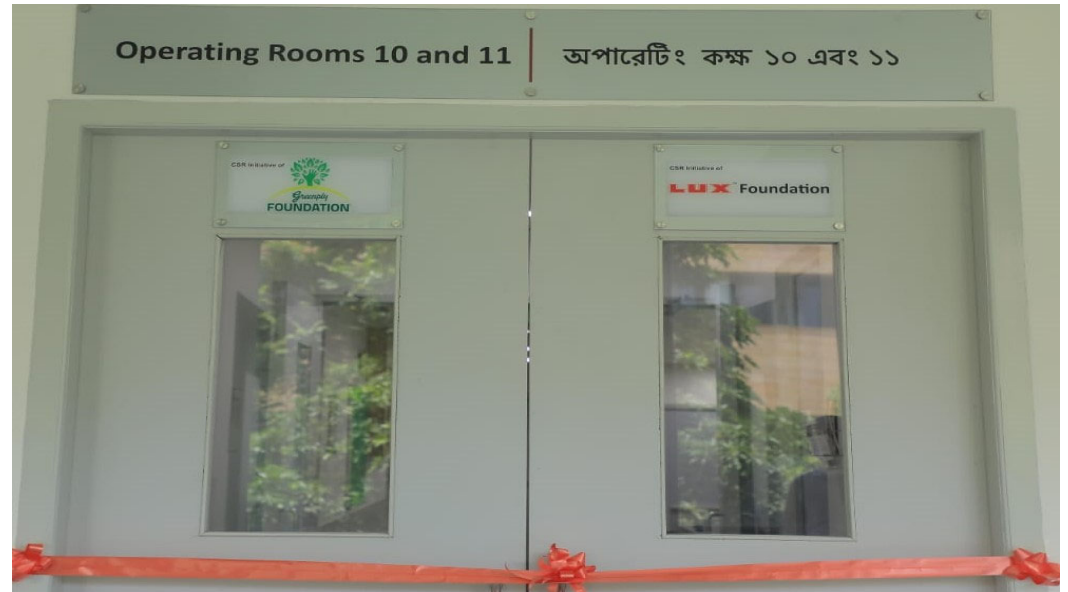
Tata Medical Center Operation Theatre
