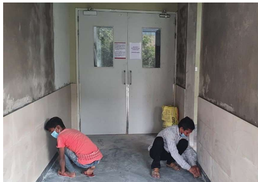
Tata Medical Center Operation Theatre - Construction
