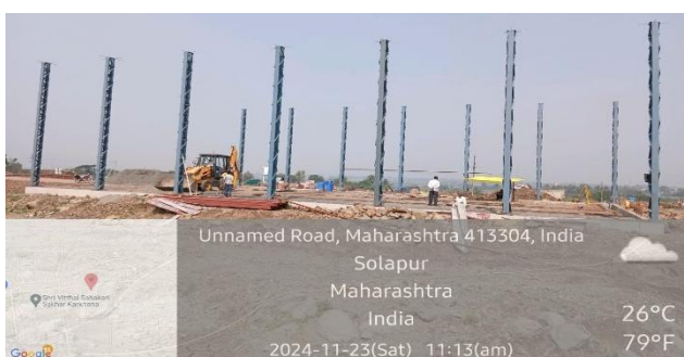
Mechanical Work at CBG Plant
