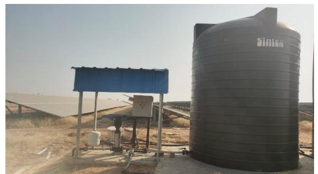
Pumping System with Water Storage
