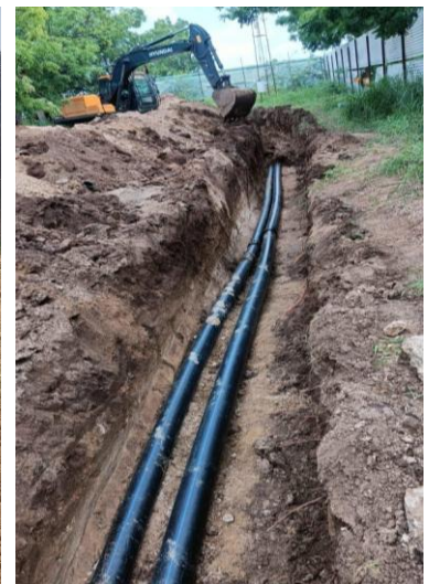
Laying of Pipe
