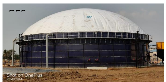
GFS Digester Tank (Completed)
