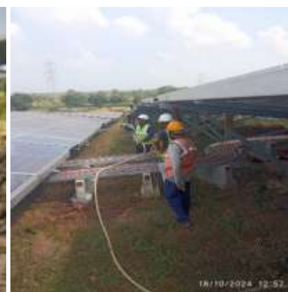
Solar Module Cleaning
