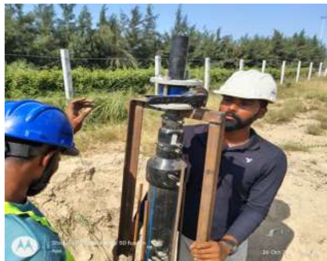
Joining Pipes and Other Related Fittings
