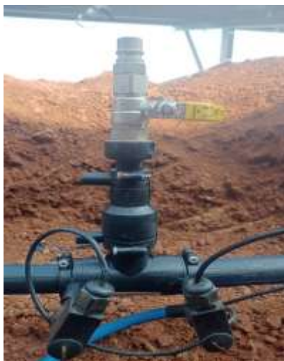
Electrofusion Jointing
