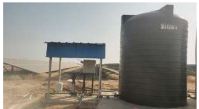
Pumping System with Water Storage
