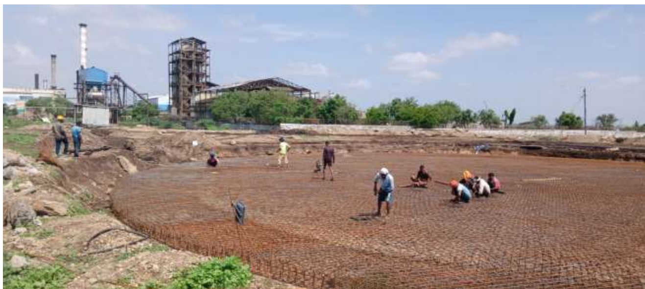
Compressed Bio Gas (CBG) Digester Raft
