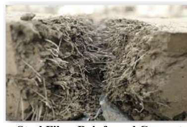
Steel Fiber Reinforced Concrete Flooring
