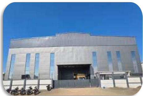
Unit-III Shendra, Aurangabad Registered Office
