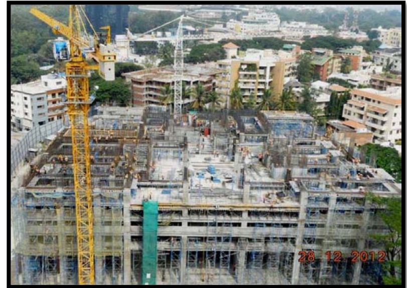
Current Construction Progress
