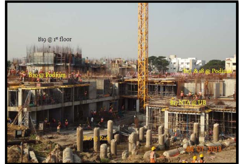
Current Construction Progress
