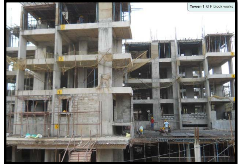
Current Construction Progress
