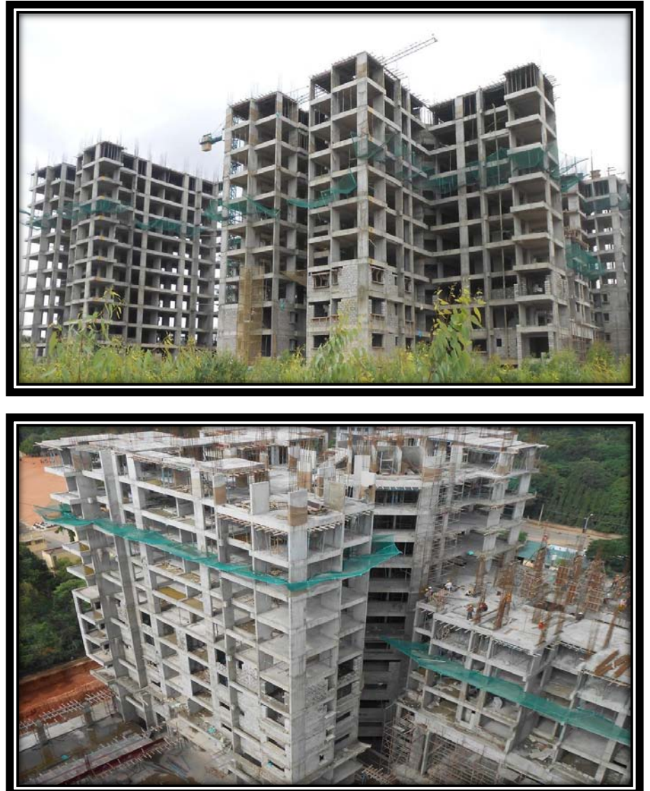
Current Construction Progress
