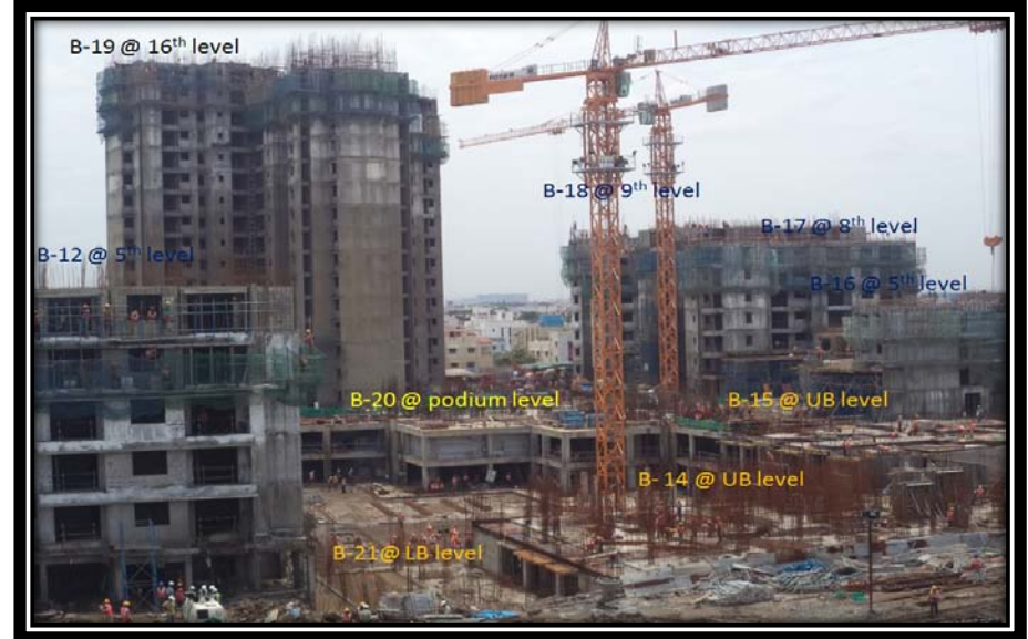
Current Construction Progress
