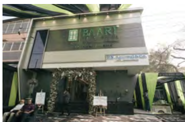
Experience centre, Jodhpur
