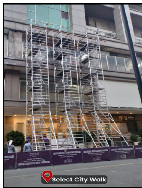
Rental supply of Aluminium Scaffolding (Model MST125-06 and 2.5m Bridge Sections) at Select City Walk Mall, Saket, New Delhi
