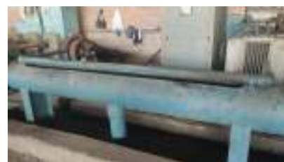
Cooling Part of Tube Mill
