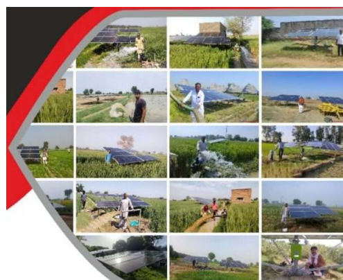
Solar Water Pump Installations in the Field
