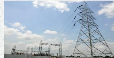
Tower & Substation EPC
