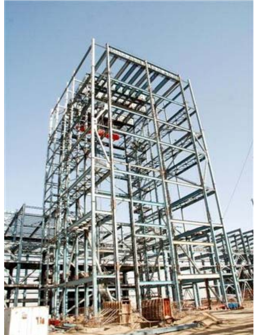
Boiler Structure 1 with drum
