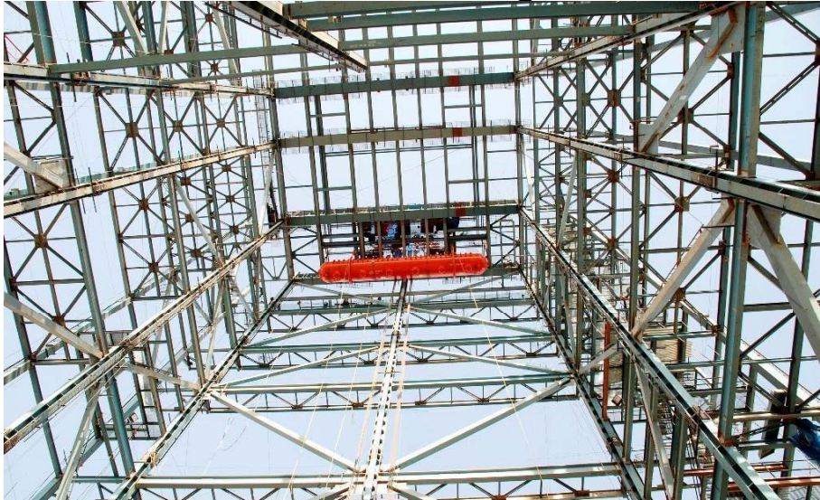
Boiler Structure 1 with drum
