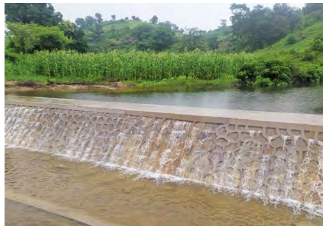
Water harvesting structure (check dam/anicut) created in Udaipur, a water scarce region in south Rajasthan
