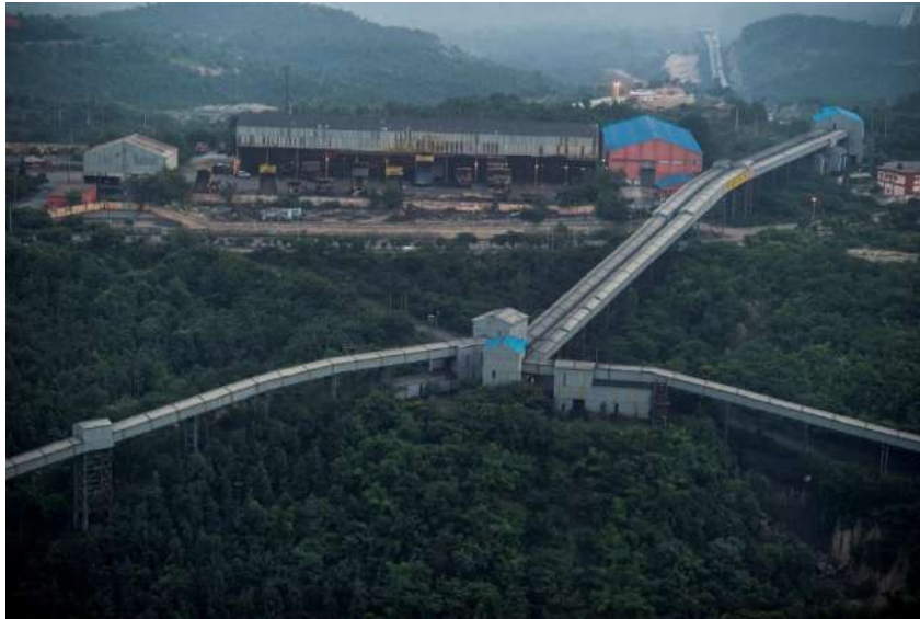
Fig. 50-Plantation around conveyor roads
