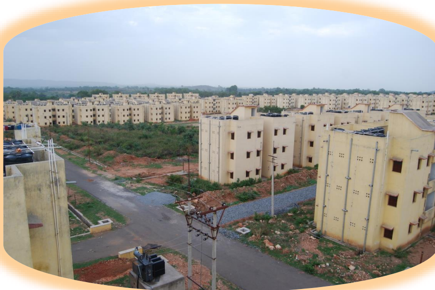
Fig. 26 - Rehabilitation site in BCCL
