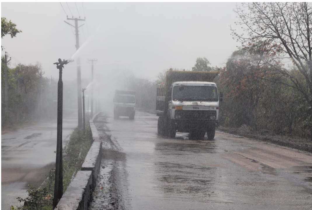
Fig. 45 - Water sprinkling in Coal Transport Roadways
