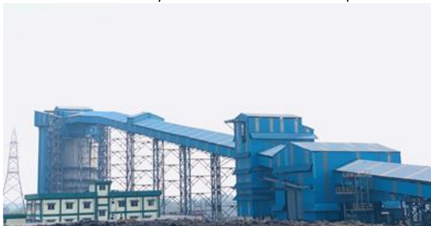
Fig. 36 - Silo in Lingaraj OCP of MCL
