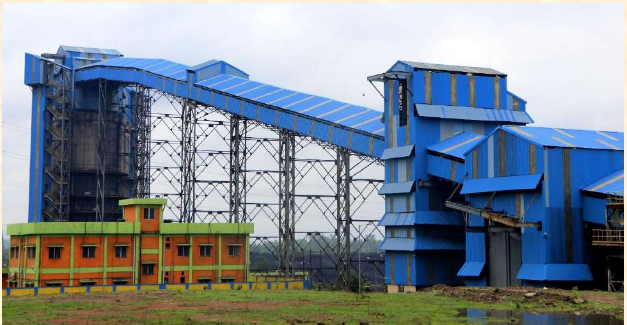
Fig. 17 - Silo in Lingaraj OCP of MCL
