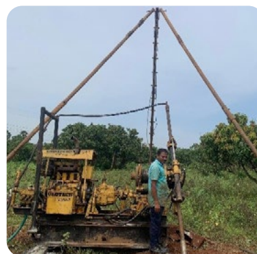
● Core drilling machines deployed at Samalpatti Rare Earth Element (REE) block
