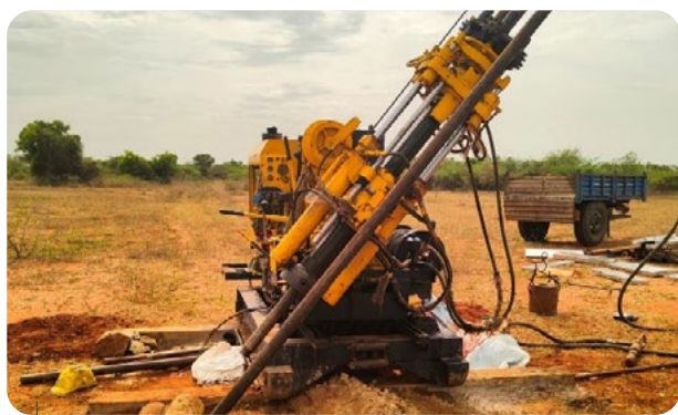
● Core drilling machines deployed at Arasanuru Graphite Block
