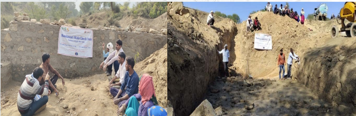
Check dams being constructed in Alwar district to catch and channelize rain water. Another sustainable initiative is to channelize and save water through a project of "Water conservation through installation of rainwater harvesting structures in the form of check dams and gabion structures" in Alwar, Rajasthan. PFS has funded four check dams and two gabion structures to improve ground water situation in the area.
