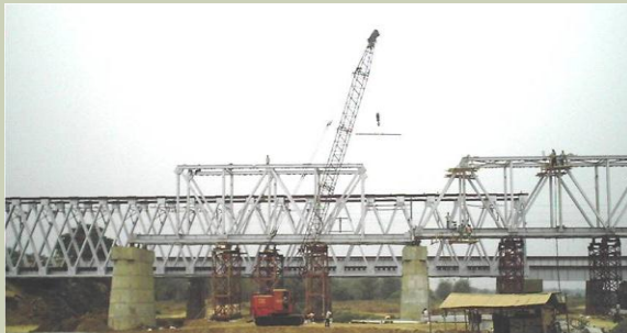
Construction of washed away Bridge No. 168 on Howrah – Chennai main line for South Eastern Railway – restoration work as well as permanent bridge was completed in 8 months
