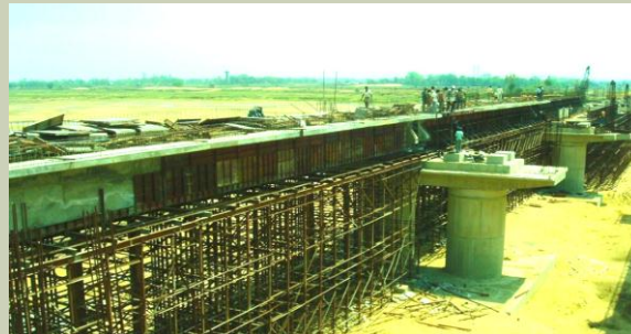
Work in progress for Bridge over River Ajoy consisting of 32 nos. 30.5m span PSC box girders for 2-lane traffic. Foundation consists of 1.2m dia piles.
