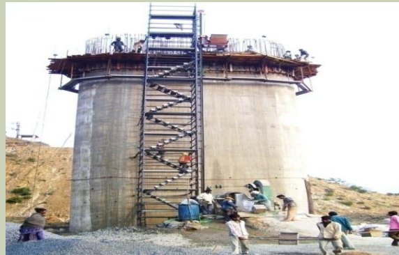
Pier casting in progress with slip-form shuttering at Barakar Rail Bridge project. Pier heights range from 17 to 27m and casting of full height is completed in 7-10 days.
