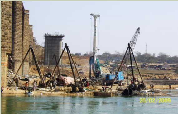
Piling work in progress at Barakar Bridge site for Eastern Railway. 1.5m and 1.2m dia piles were constructed with rotary and conventional rigs and anchored more than 6m in hard rock.
