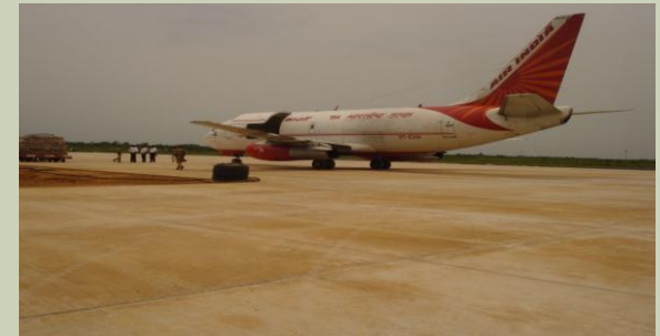
Completed apron with pavement quality concrete at Agartala Airport for Airports Authority of India
