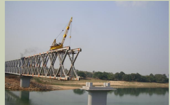
Cantilever launching of 92m span in progress for Rail Bridge over River Mahanadi at Naraj, Cuttack
