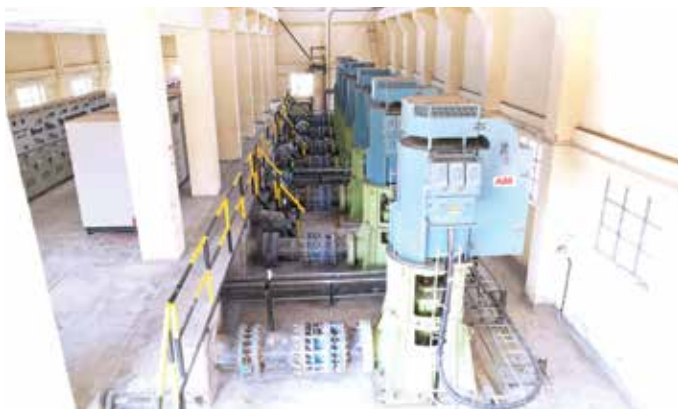
Installation of Pumping Machines 1350 KW Capacity each VT Pump 6 Nos for Minor Irrigation and Ground Water Development Division, Koppal, Kushtagi, Karnataka.
