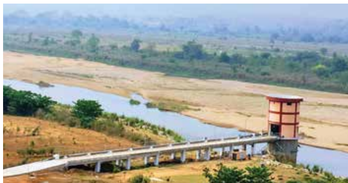
Intake Well cum Pump House at Palsing Village, Kasinagar for Gajapati Water Supply Scheme in Odisha.
