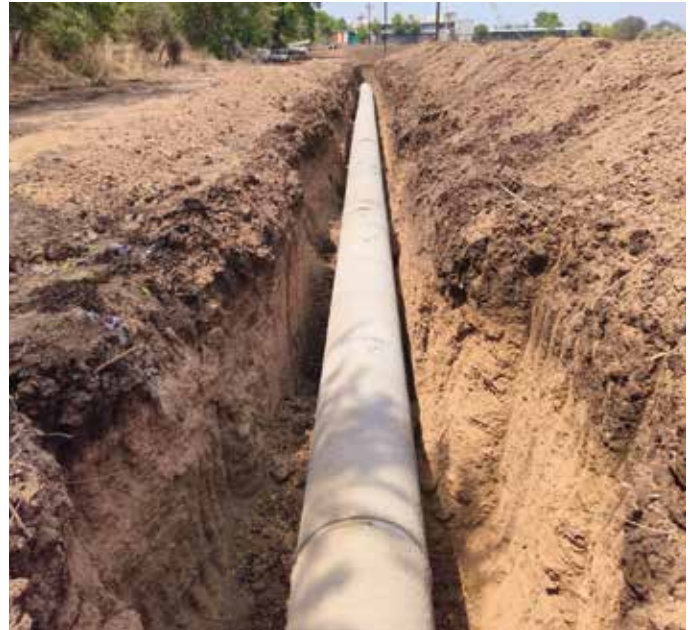
600 mm dia PCCP pipe line laying for Jalgaon Jamod and 150 villages Regional Rural Water Supply Scheme for Maharashtra Jeevan Pradhikaran in Maharashtra.
