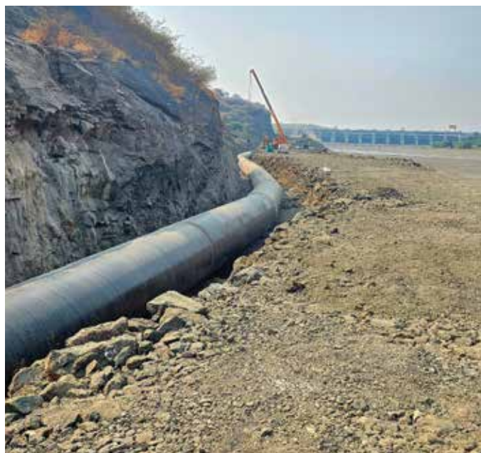
1900 mm dia M.S. pipe line laying for Varkhede Londhe Irrigation Project in Maharashtra.
