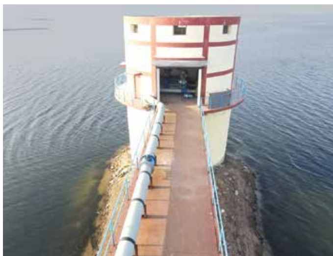
Intake Well cum Pump House at Saprar Dam for Kuraicha Water Supply Scheme in Uttar Pradesh.
