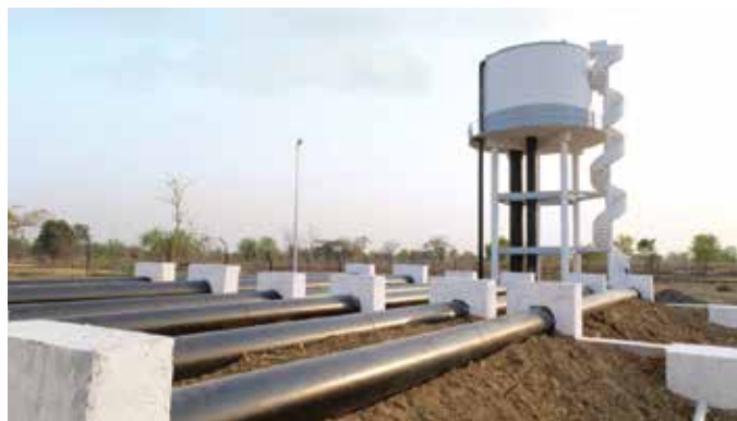
Delivery Chambers for Pauni Lift Irrigation Scheme in Maharashtra.
