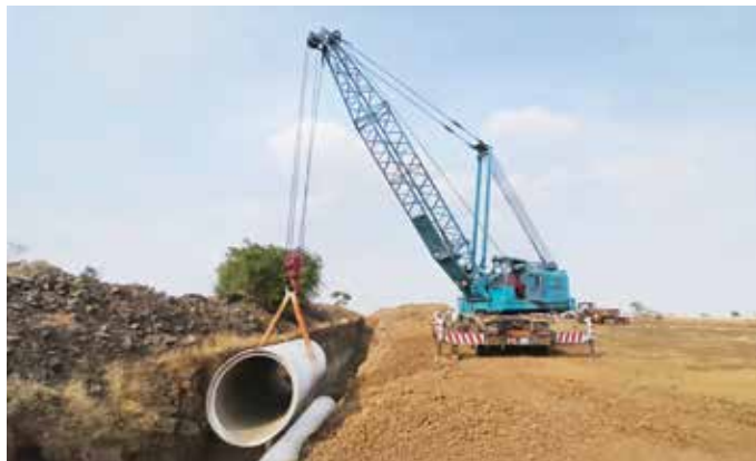
1600 mm dia PCCP pipe line laying for Man Canal of Urmodi Irrigation Project in Maharashtra.
