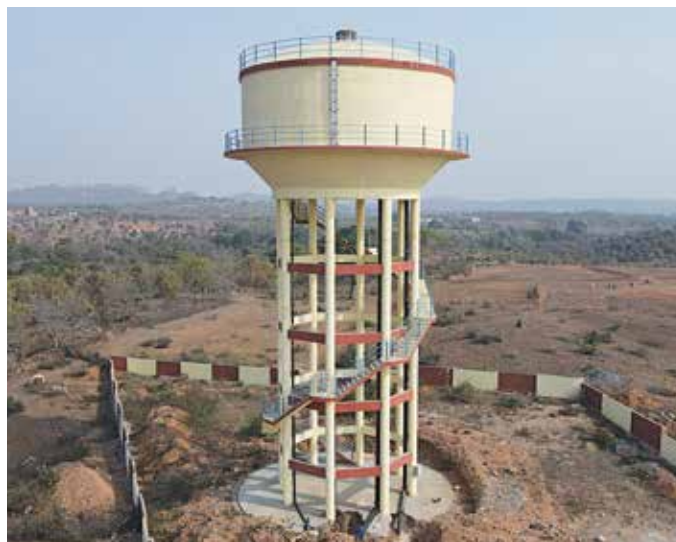
450 KL Capacity x 18 Mtr staging Elevated Service Reservoir at Kathera Rural Village for Kuraicha Water Supply Scheme in Uttar Pradesh.
