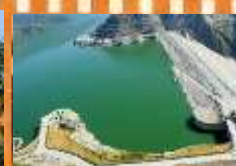
Tihri Dam, Uttaranchal
