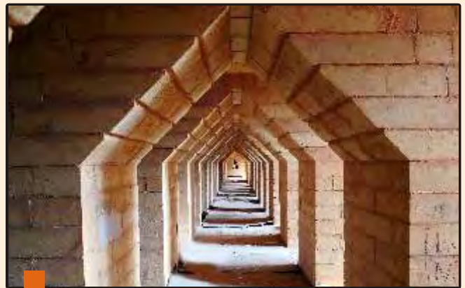
Coke Oven Flue Tunnel
