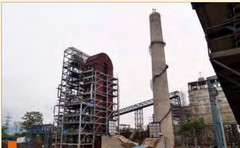
Waste Heat Recovery Boiler under construction
