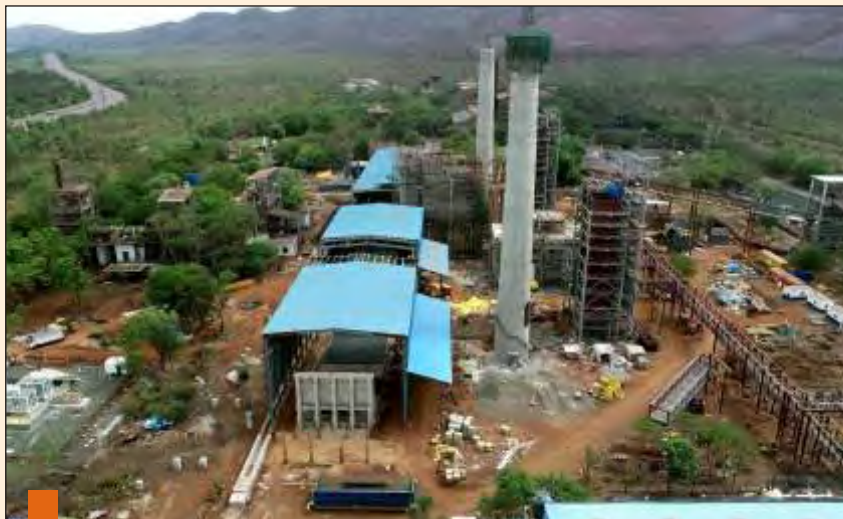
Coke Oven Plant under construction
