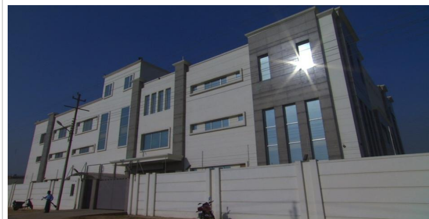
Sector 63 Noida Facility
