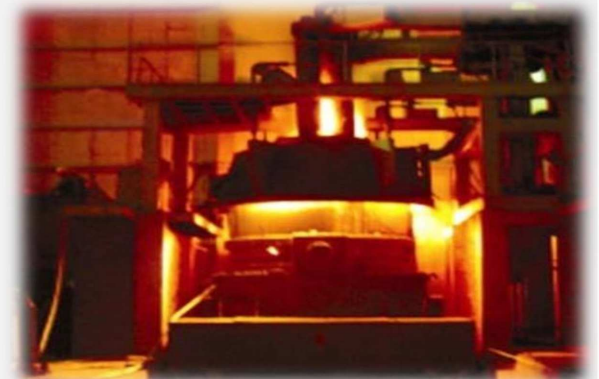
Two Ladle Refining Furnace
