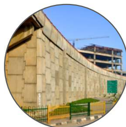
Reinforced Earth Walls
