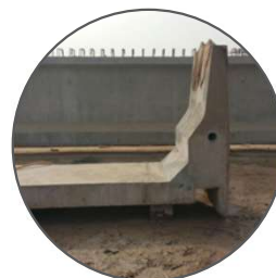
Fabricated Casting Panels and Moulds
