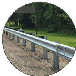
Metal Beam Crash Barrier
