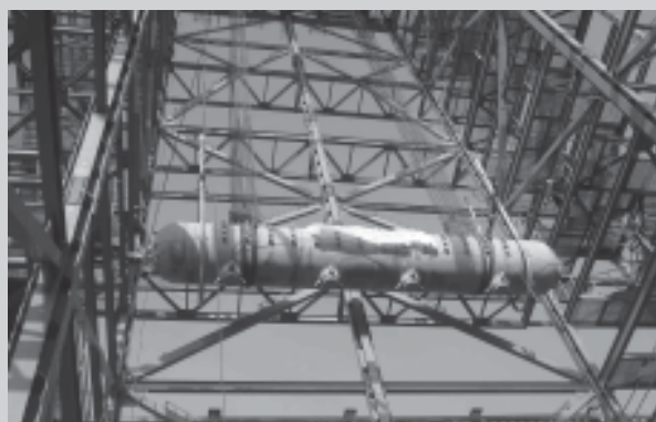
Boiler Drum Lifting at 4x125 MW STG based Project at Kosti, Sudan
