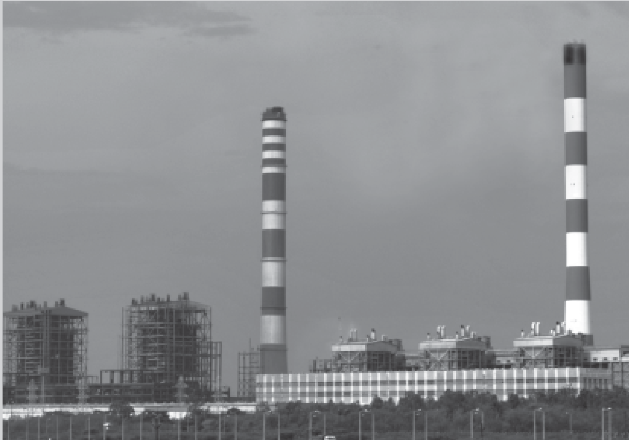
2x600 MW North Chennai TPS by BHEL on EPS basis, equipped with country's first large capacity new series Turbo-Generators
