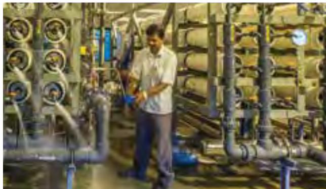
RO membranes of RODM plant commissioned by BHEL at RPCL Yeramarus
