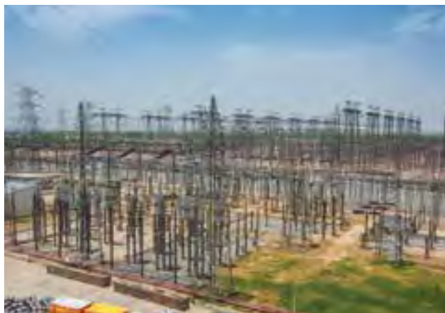
400 kV AC yard for HVDC Agra converter station
