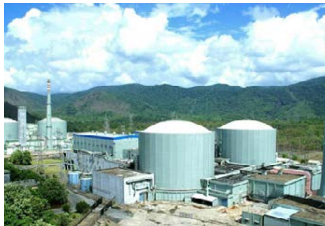
Kaiga Nuclear Power Plant in Karnataka is equipped with BHEL manufactured Turbine-Generator sets
