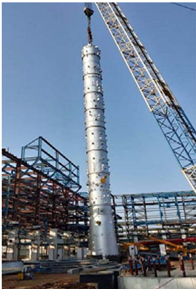
Sour water stripper Stage – N column at Vishakhapatnam, under commissioning by BHEL
