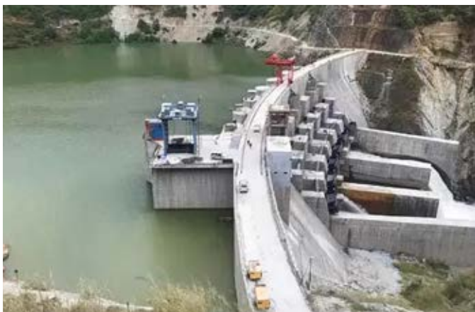
4x150 MW Kameng HEP commissioned by BHEL in Arunachal Pradesh, the highest rating hydroelectric set in the state
