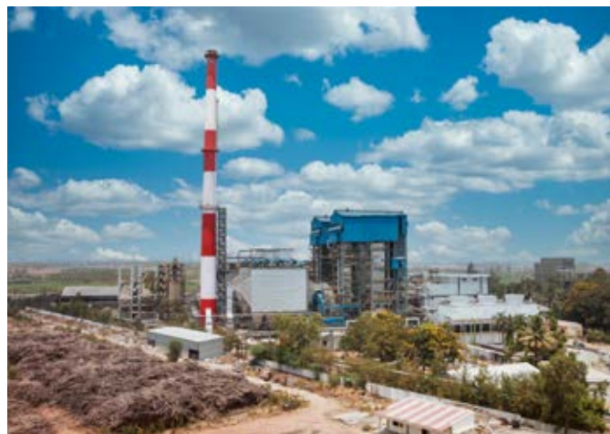
1x120 MW Grasim Harihar Captive Plant in Karnataka commissioned by BHEL
