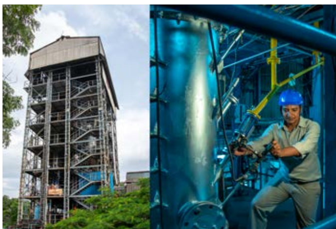
BHEL developed coal gasification facility at Hyderabad
