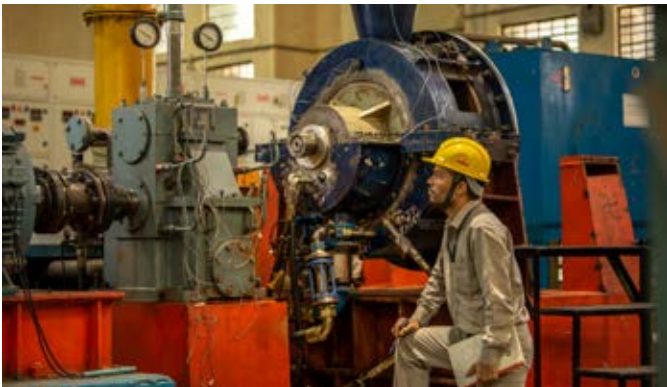
Facility for testing and rating of pumps and compressors at Corporate R&D, Hyderabad
