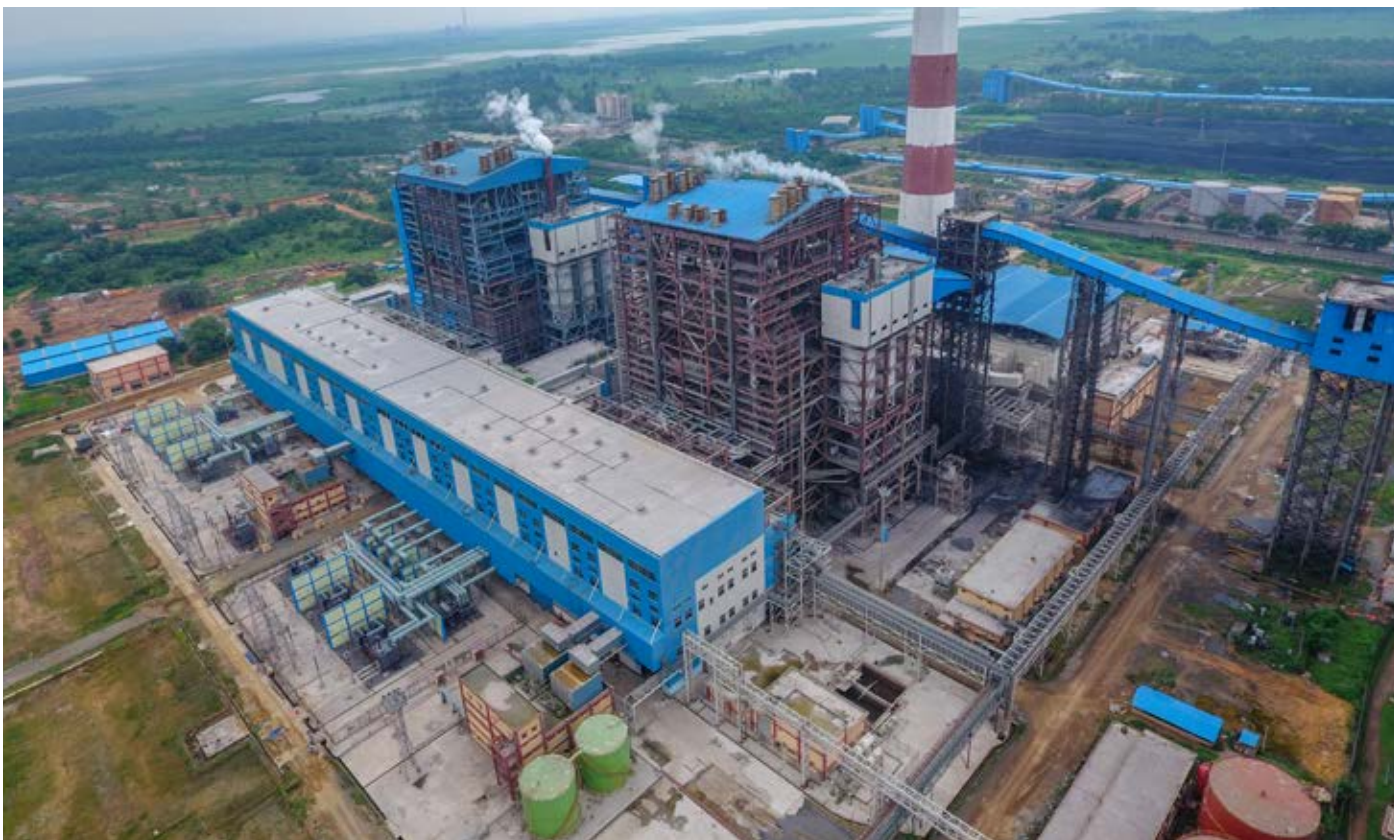
2x660 MW IB Valley Thermal Power Station commissioned by BHEL in Odisha
