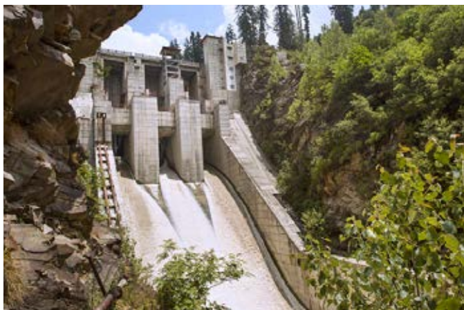
BHEL has successfully commissioned all four units of the 4X130 MW Parbati HEP in Himachal Pradesh
