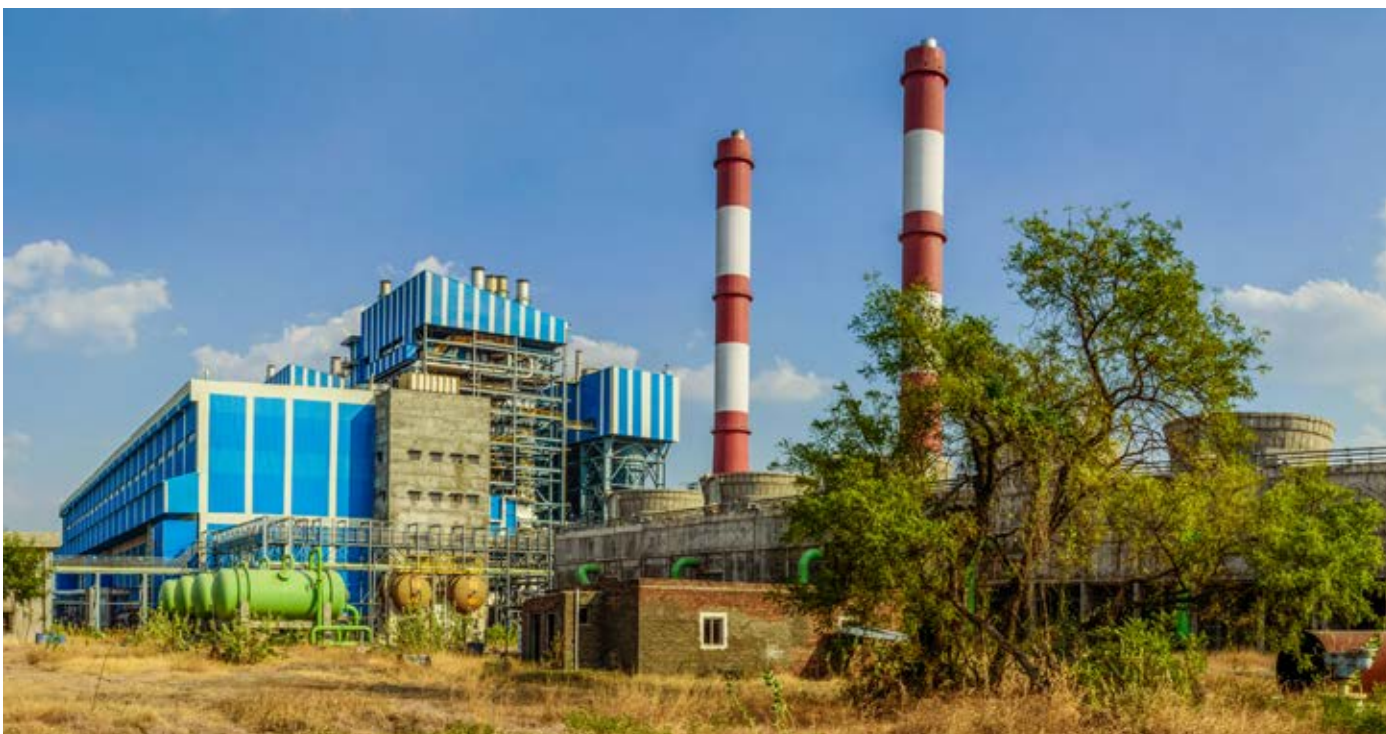
2x150 MW Sintex-Dhule Captive Power project commissioned by BHEL in Maharashtra
