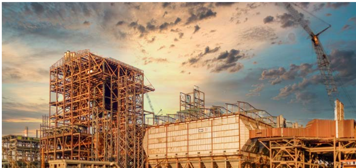
A typical supercritical power plant under erection. BHEL currently has over 150 ongoing projects all over the country.
