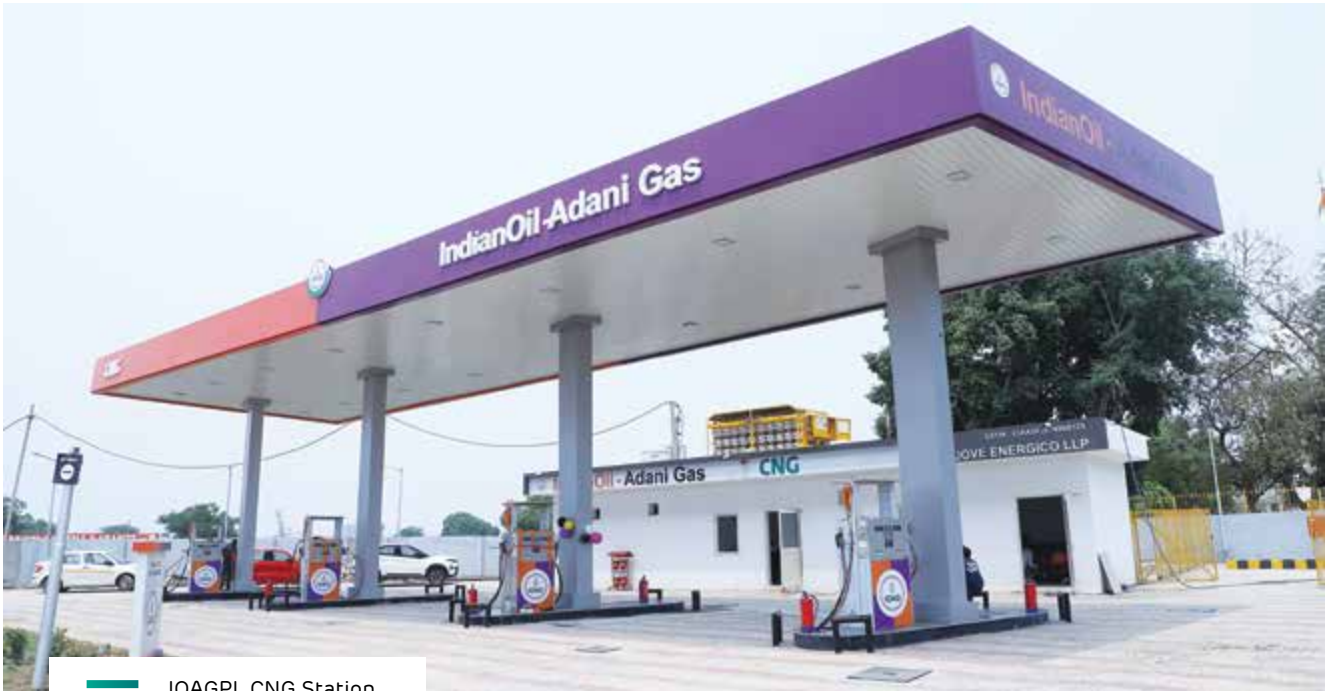
IOAGPL CNG Station
