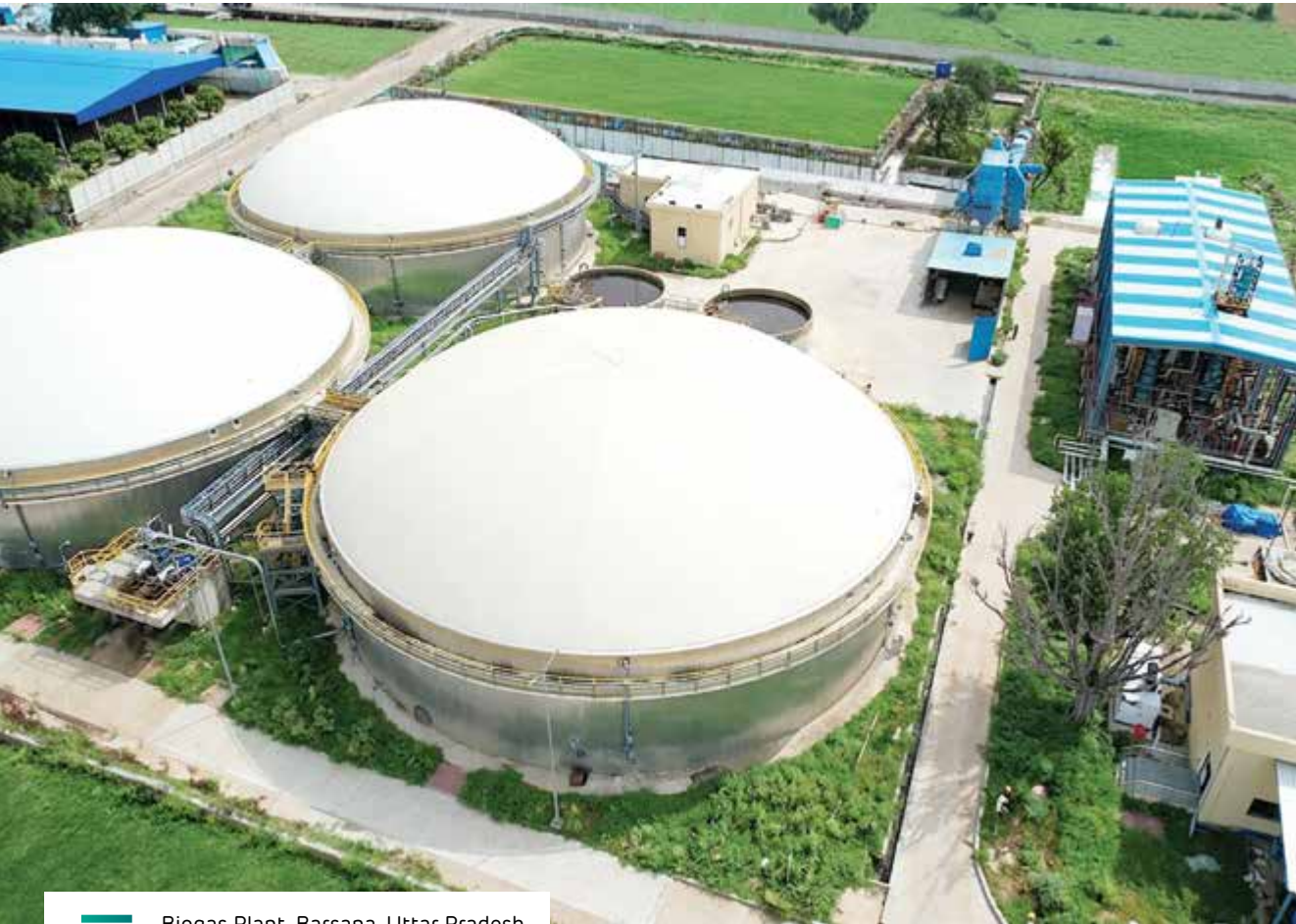
Biogas Plant, Barsana, Uttar Pradesh
