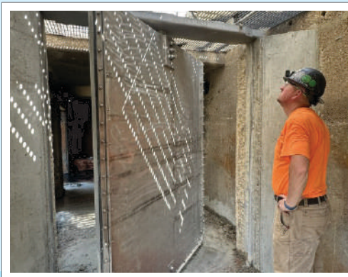
Installation of butterfly gate at bissell point wastewater treatment facility, USA
