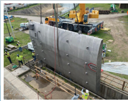
Shockoe diversion structure improvement, USA Stainless steel crest gates (Actual Site)
