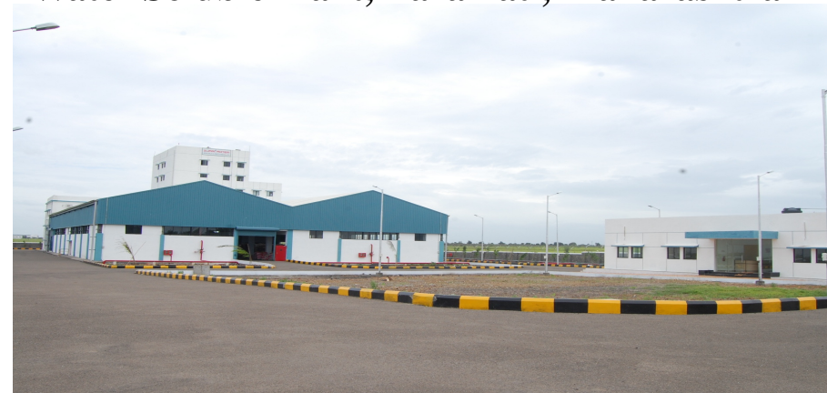
Water Soluble Plant, Baramati, Maharashtra
