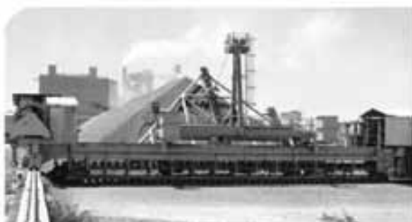
BRIDGE TYPE SCRAPER RECLAIMER
