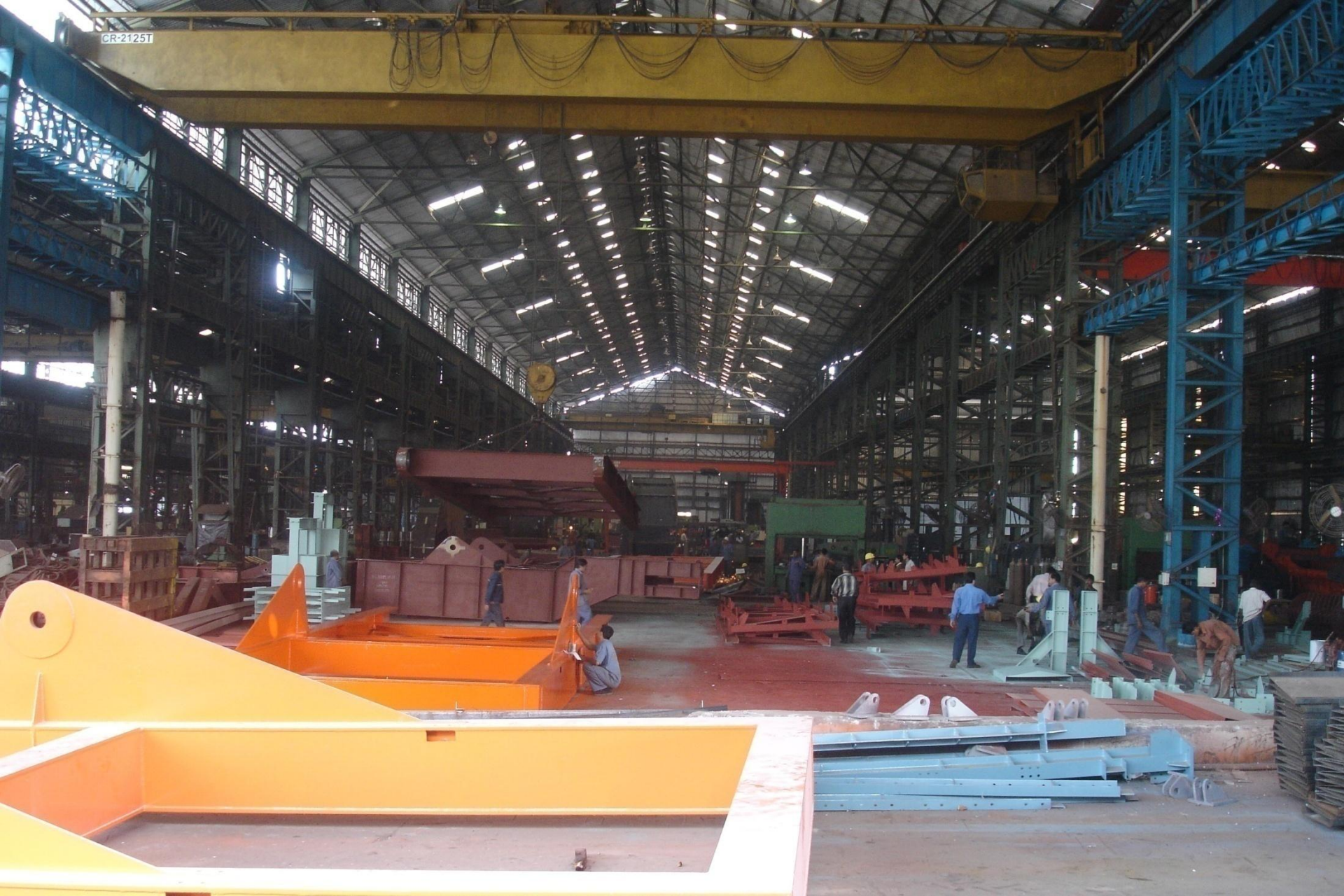
Manufacturing activities in the Heavy Fabrication Shop
