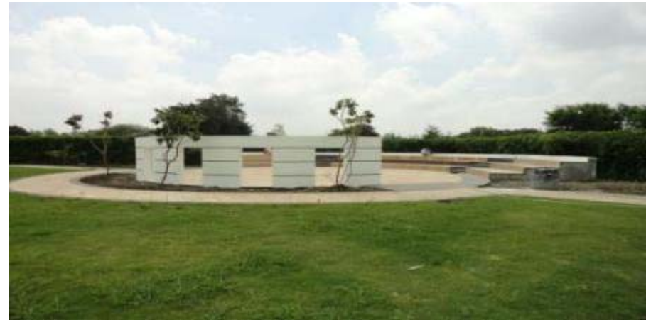
Club House & Swimming Pool
