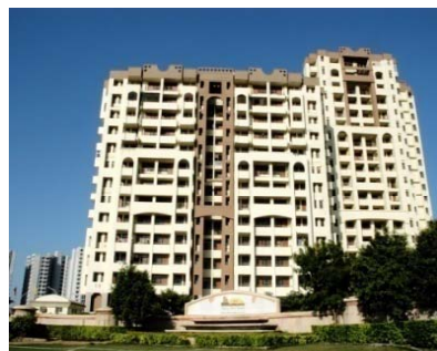
Valley View Estate, Gurgaon
