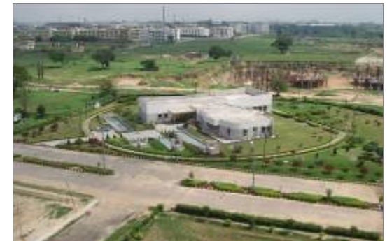
Actual photograph of the project
