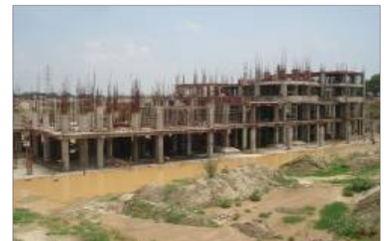
Actual photograph of the project
