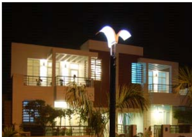
Actual photograph of the project
