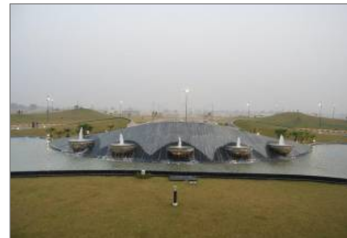
Actual photograph of the project
