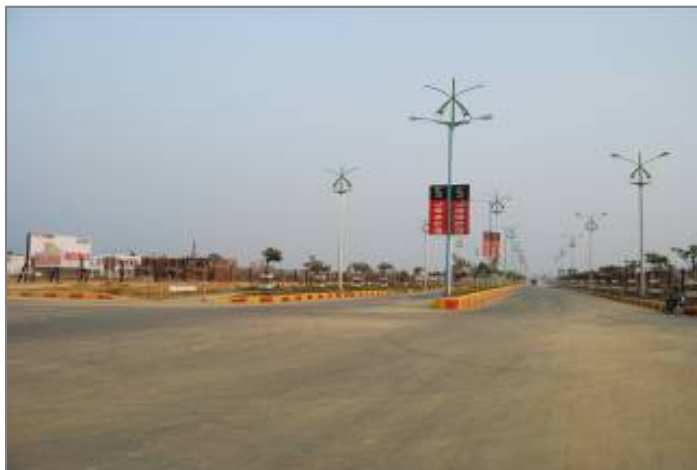
Actual photograph of the project
