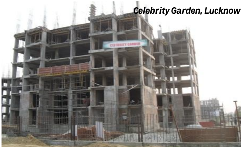
GHS under construction ~187,705 sq.ft.
