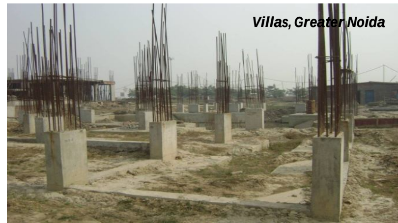
Low-Rise Built-Ups under construction ~874,335 sq.ft.
