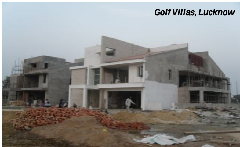
Low-Rise Built-Ups under construction ~1,899,444 sq.ft.
