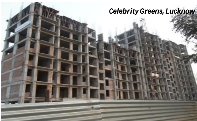
GHS under construction ~160,261 sq.ft.
