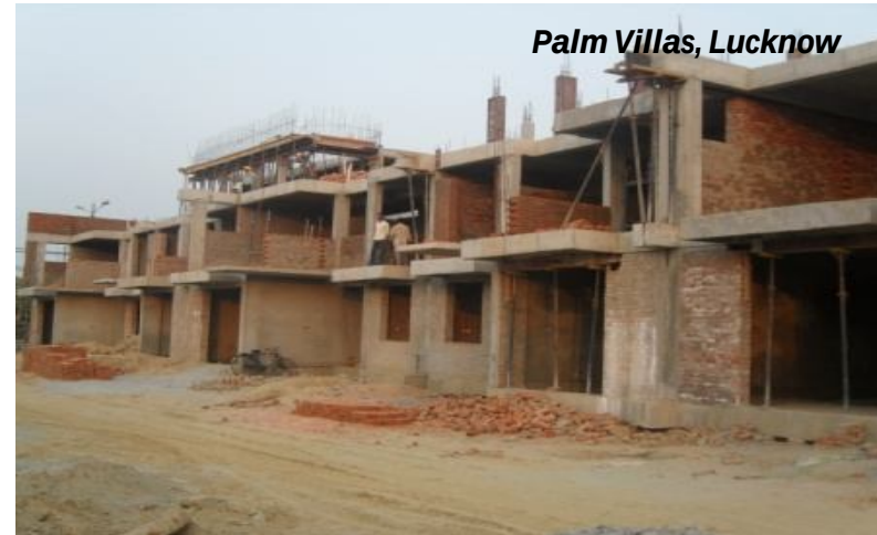
Low-Rise Built-Up under construction ~347,472 sq.ft.
