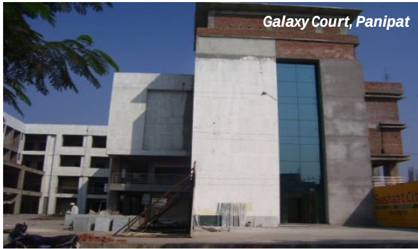
Commercial under construction ~194,111 sq.ft.
