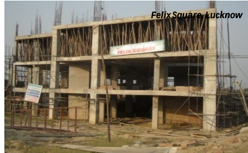
Commercial under construction ~165,945 sq.ft.
