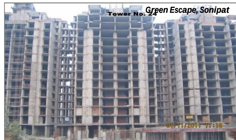
GHS under construction ~2,320,346 sq.ft.
