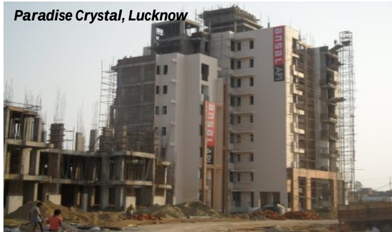
GHS under construction ~303,777 sq.ft.
