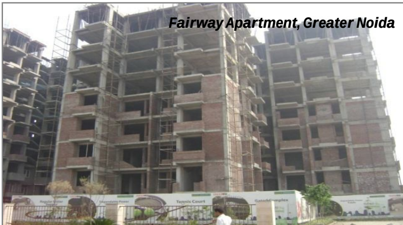
GHS under construction ~1,287,551 sq.ft.
