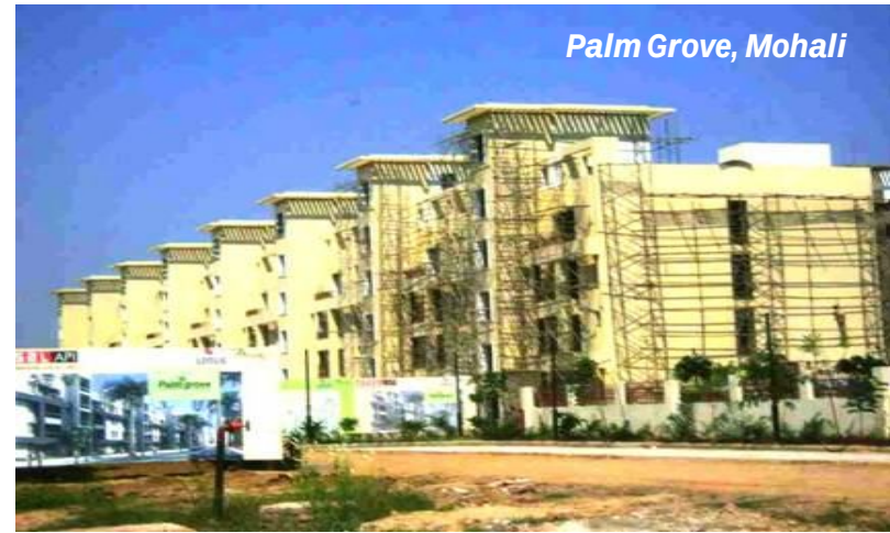
GHS under construction ~195,200 sq.ft.
