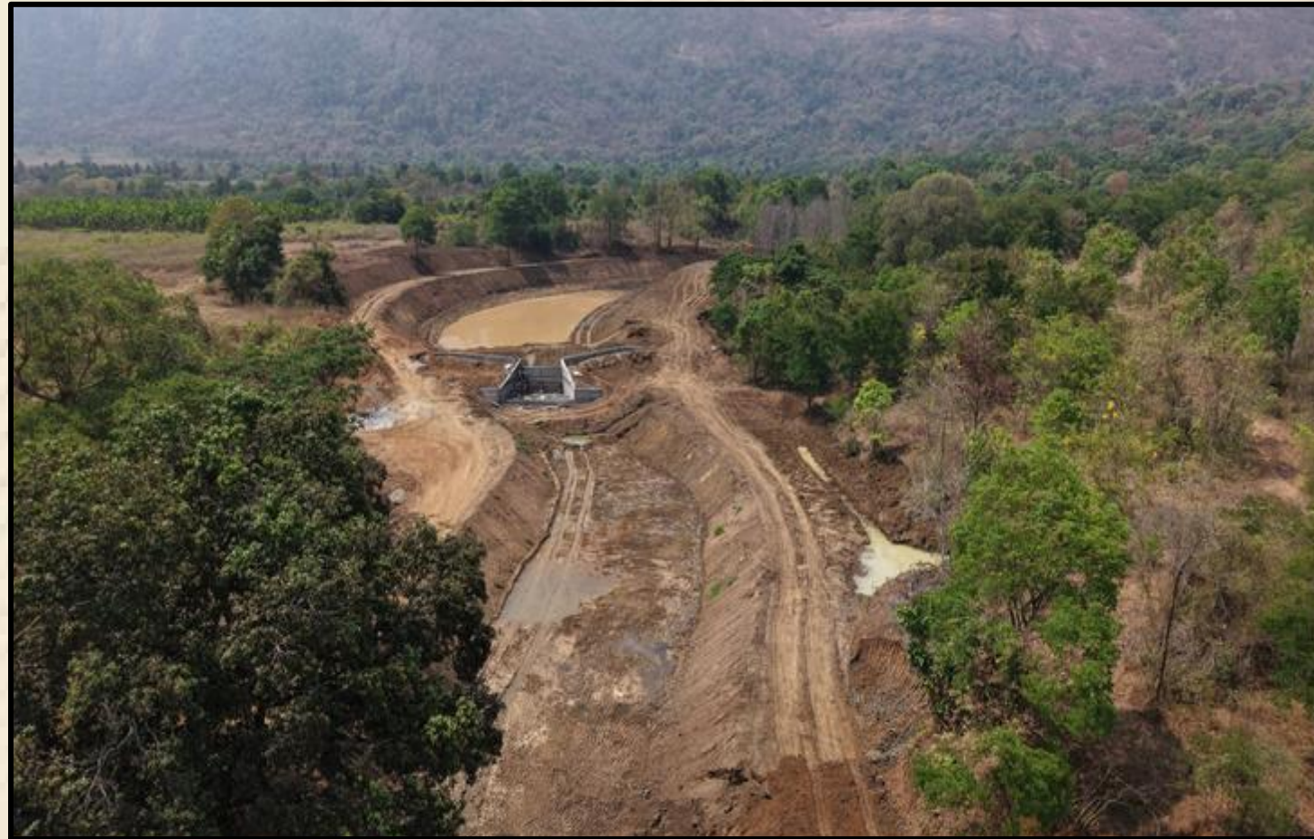
➤ Water Augmentation Beyond the Fence – Checkdam Restoration -
