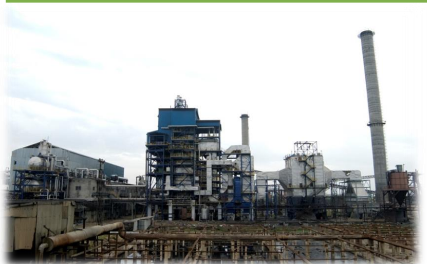
Power Generation yards, ESPs and Flue Stacks
