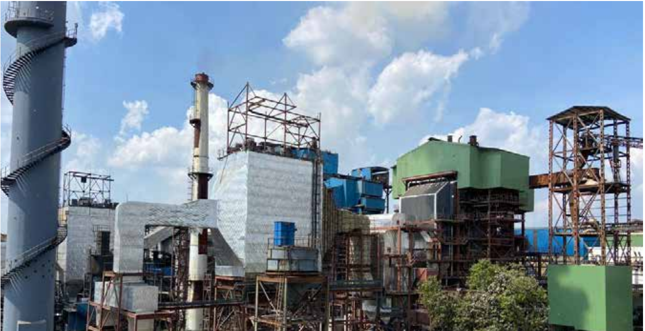
Cogeneration Plant at Haliyal
