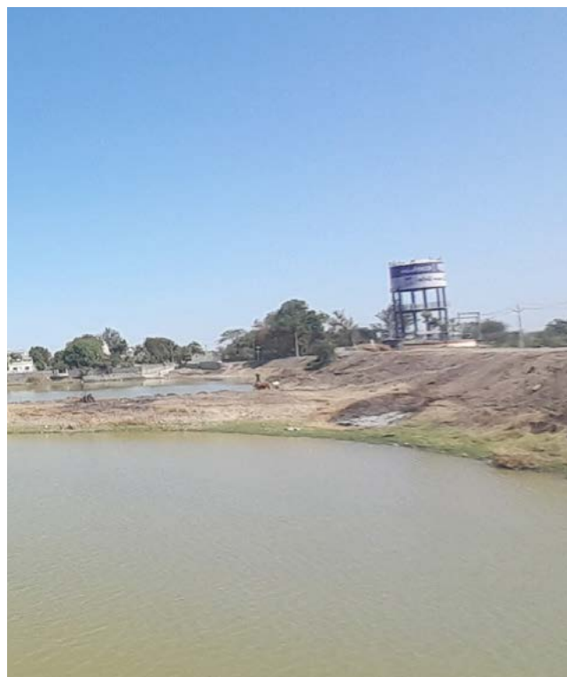
— Deepening of Pond at Akhod Village, to enhance groundwater availability
