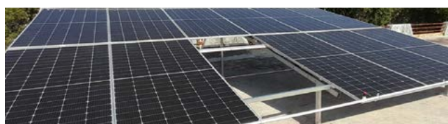
— Solar Panel Installation at Karakhadi High School, Vadodara, Gujarat
