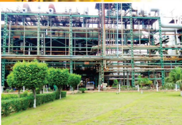
Works Location 3 : Village Karimganj, Teh. Shahabad, Distt. Rampur, Uttar Pardesh.
