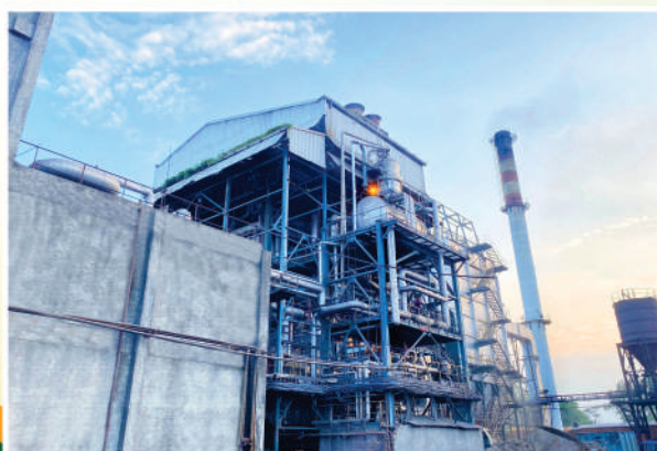
Works Location 4 : Village Lauhka, Teh. Patti, Distt. Tarn Taran, Punjab.
